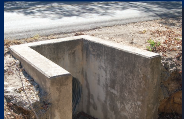
Drainage structure very near roadway edge
