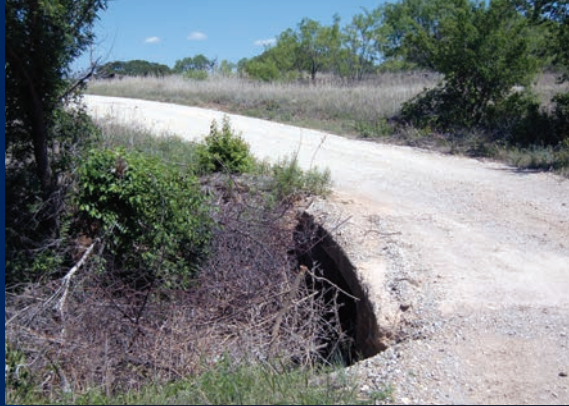
Drainage structure on curve at edge of unpaved road
