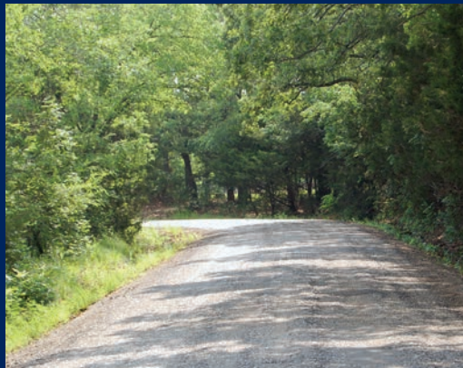
Very limited sight distance around sharp turns
