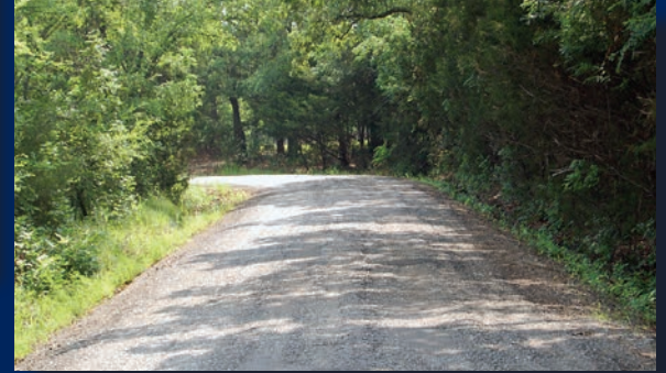
No warning or marking of sharp turn
