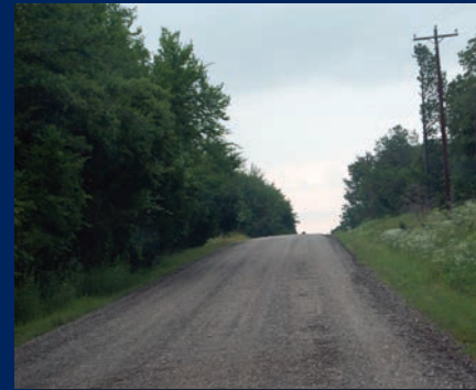
Sight distance over hill may be incompatible with speed accommodated by surface.
