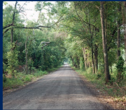
Narrow ROW – Trees very near roadway edge
