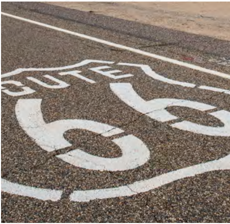
Large route shield markings like these should be used in advance of major freeway junctions to guide drivers to the correct lane.
