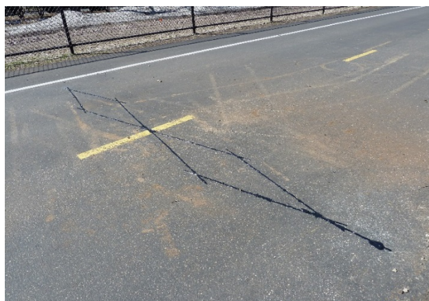
Figure 16: Calibration Performed before Sealing the Saw Cut to Ensure Proper Performance
