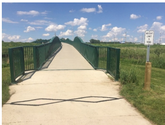
Figure 21: Infrared and Short Duration Inductive Loop Installation on Surface of a Shared-use Path
